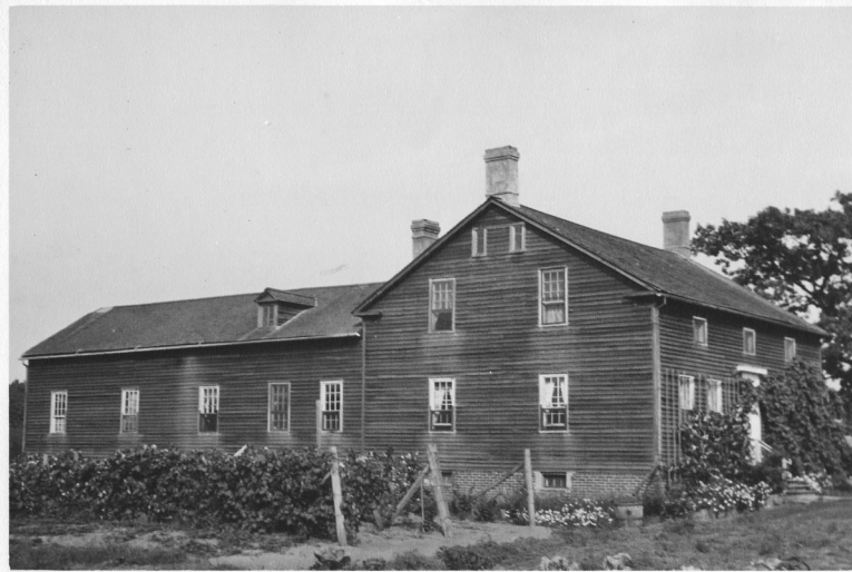
Above-grade basement windows.
